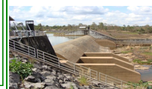
Visit Xeset 1 Dam site
