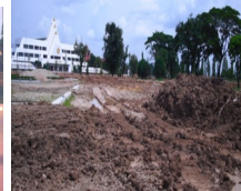
Preparing Land at park field
